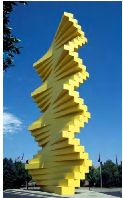
The sculpture has become a Denver icon. Constructed of 33 pre-fabricated concrete elements, the wall is held together through the center with a refueling mast taken from an aircraft carrier. Two million pounds of concrete were used to create the 85-foot tall sculpture.
