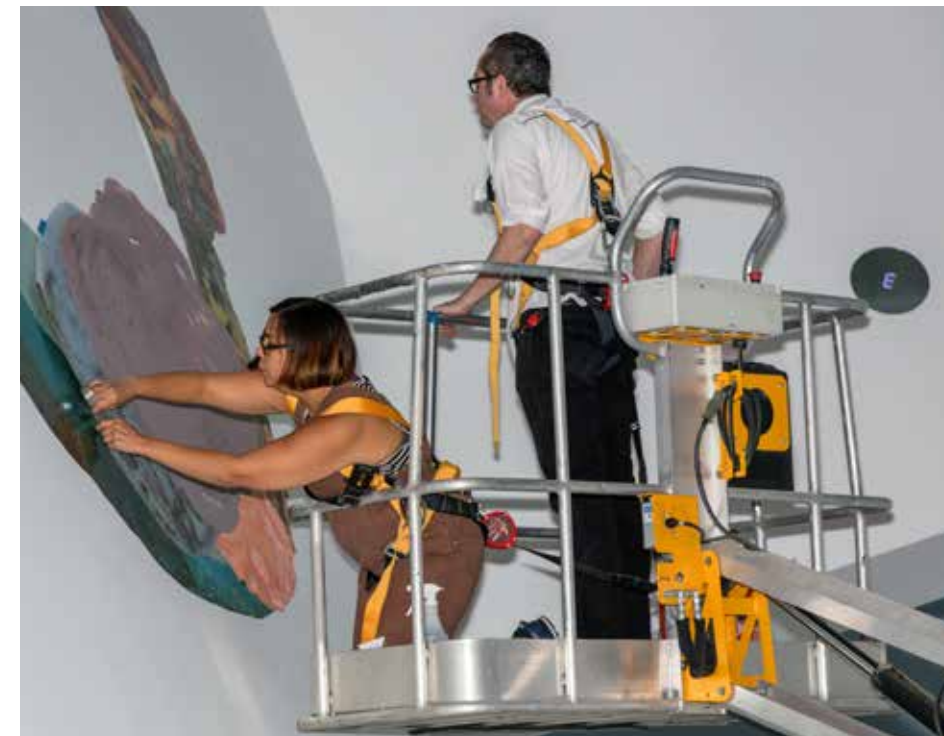
Xochi Solis and Kevin Hester, associate manager of installations, installing Solis' artwork for Mi Tierra .
