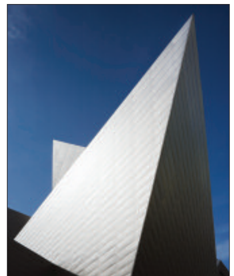
Frederic C. Hamilton Building. Photo © Jeff Goldberg.
