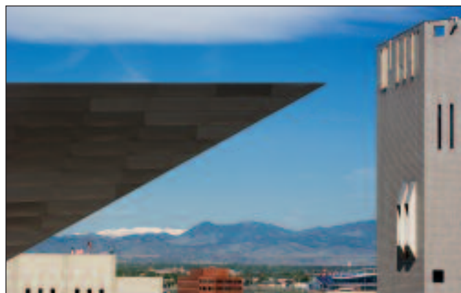
Frederic C. Hamilton Building. Photo © Jeff Goldberg.
